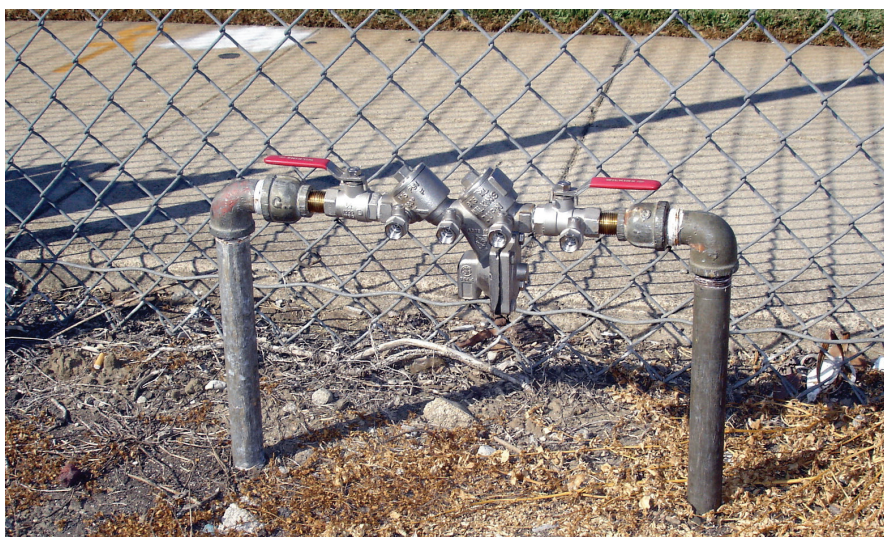
Undersized backflow preventer: 1-inch piping & 1/2-inch backflow preventer
