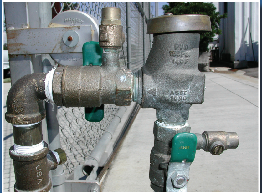
Watts PVB- Incorrect
