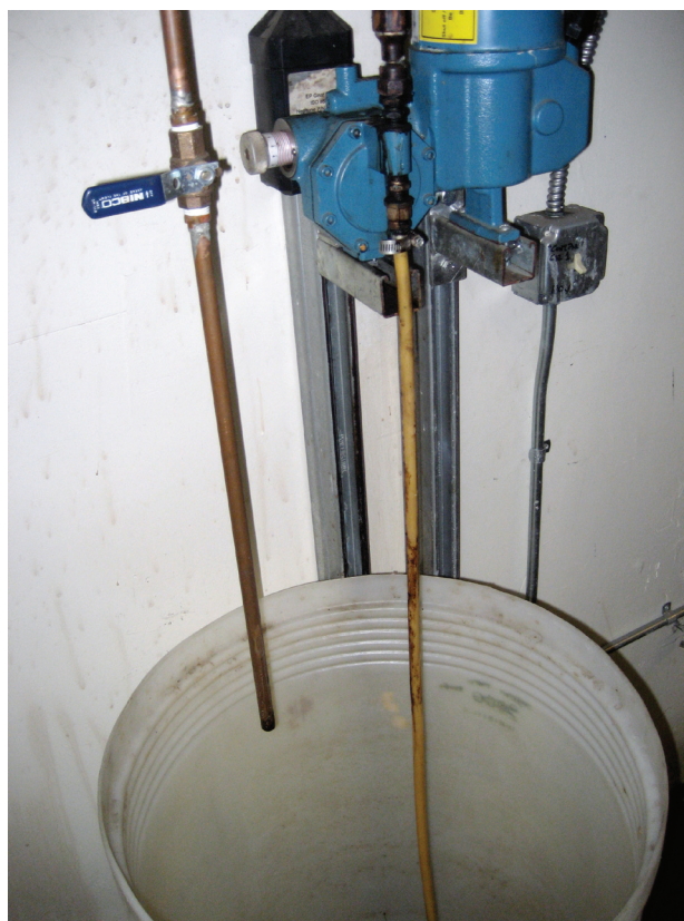
A fixed pipe with an Indirect Cross-Connection
