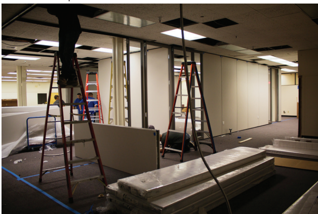
New Offices Under Construction
