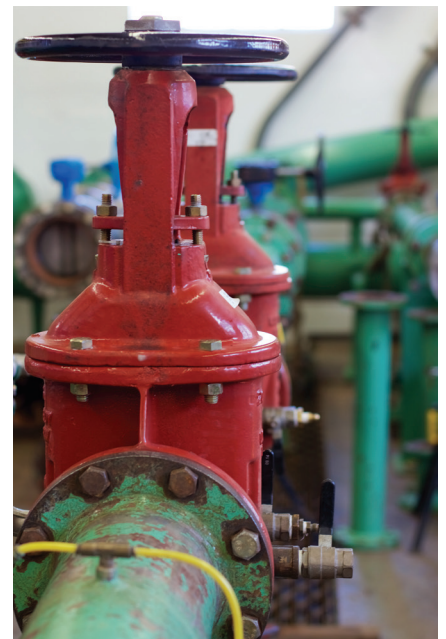
Flanged Shutoff Valve
