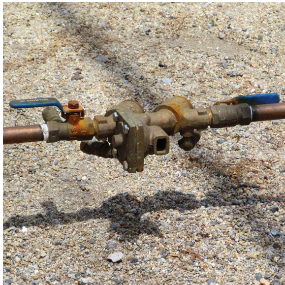
Reduced Pressure Principle Assembly (RP) rotated on its axis 90° degrees
